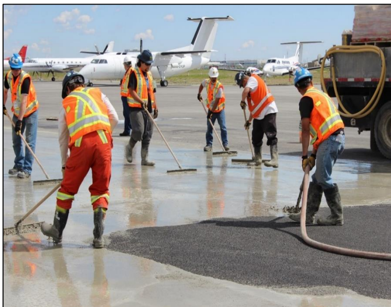
Figure 1 Pouring of cementitious grout in the porous asphalt skeleton [2].
